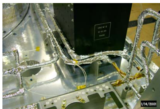
Figure 3. Pipeline covered by Multi Layer Insulation
