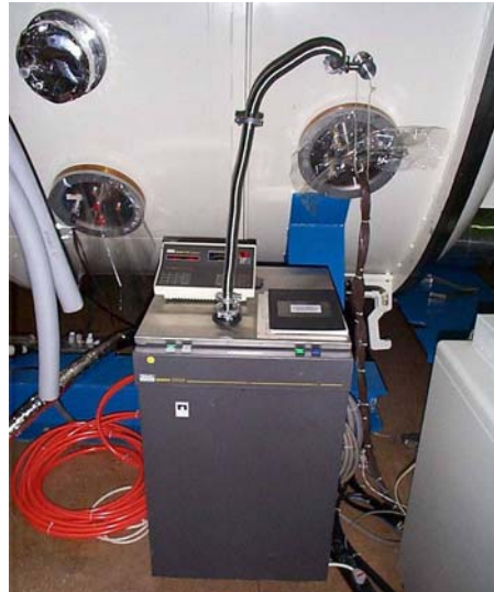
Figure 6. Leak Detector connected to TVC port
