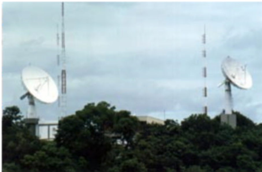
Figure 16 Antennas of Cuiabá Data Reception and Recording Station
